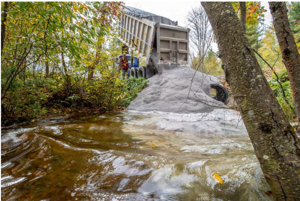
The inaugural placement of high quality limestone fines into the West Branch of Jones Run to address AMD in this headwater stream, 2018. Photo by Brett Whitling, Clarion News.
