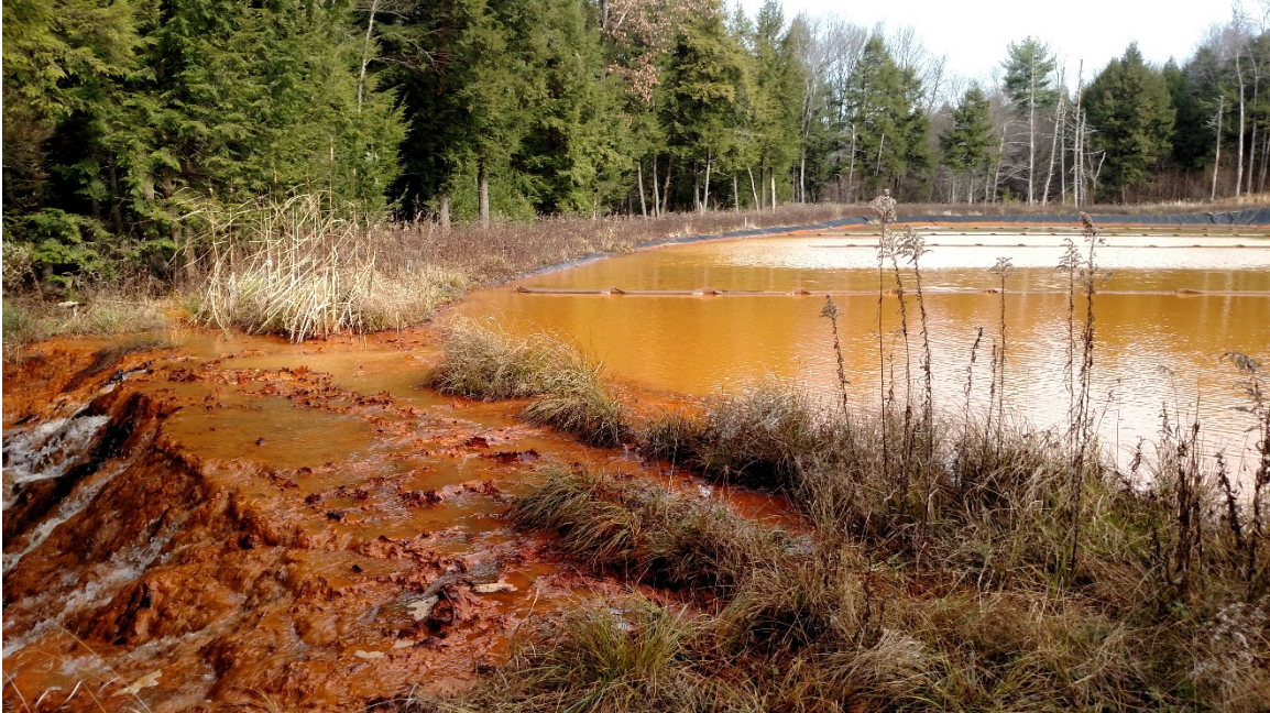
Figure 4. A clogged discharge pipe at the Markle/Kotchey treatment system causes the settling pond to discharge over the berm. Accumulated iron solids suggest the pond has been discharging in this manner for a long time.
