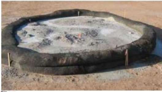
FIGURE 3.18 Typical Compost Sock Washout Installation
